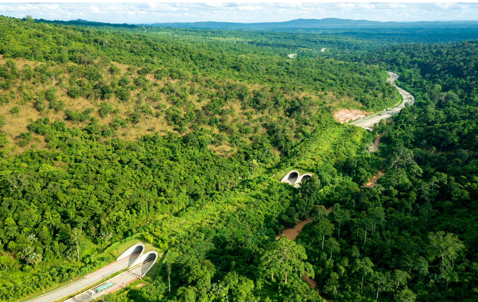
Aerial view of wildlife corridor built across road, enabling wildlife to cross safely. (Credit: thianchai siythikongsak / Contributor, Getty Images)
